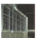
Sampling across the fresh air make-up vent can be used to prevent the introduction of external pollutants, and to prevent internal detectors from issuing false alarms.
